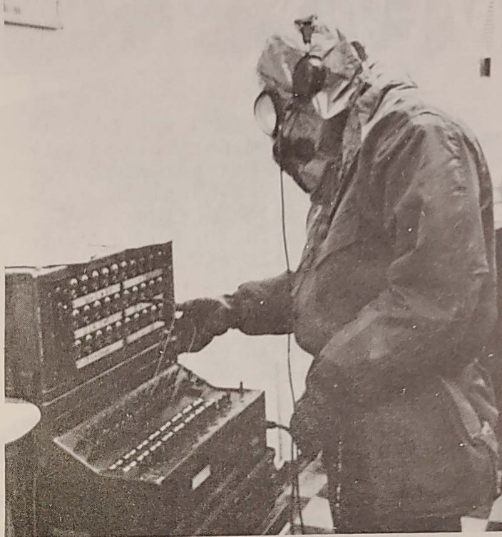
TSgt Renny Shoemaker, telephone equipment repairman for Comm Flight, checks out a switchboard while wearing full dress chemical warfare gear.
